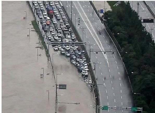
< Inundation of Olympic Expressway >
