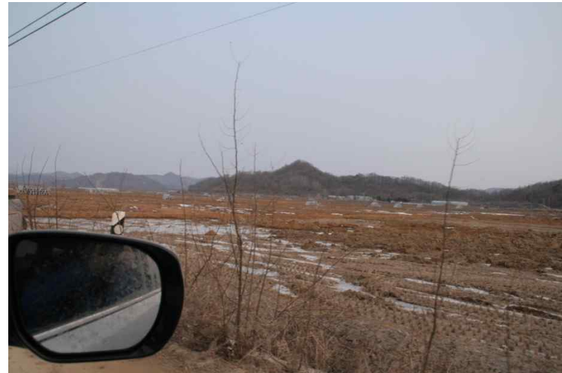
Point unit - Construction sites
