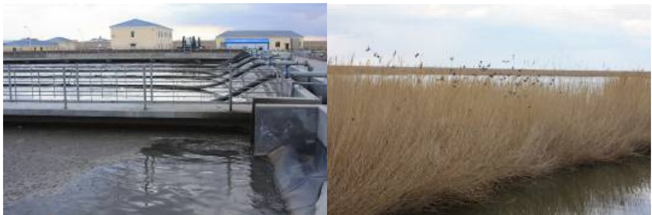
[Figure 9] Modern wastewater treatment plant and artificial wetland in Erenhot
