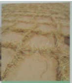
Grass Grid Sand Barrier, Naiman Banner of Inner Mongolia, China
