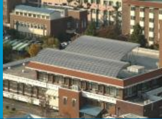
KNU Dormitory PV, 50kW
