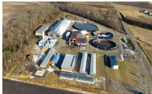
Naka-Shikaoi Biogas Plant (Source: Shikaoi Town)
