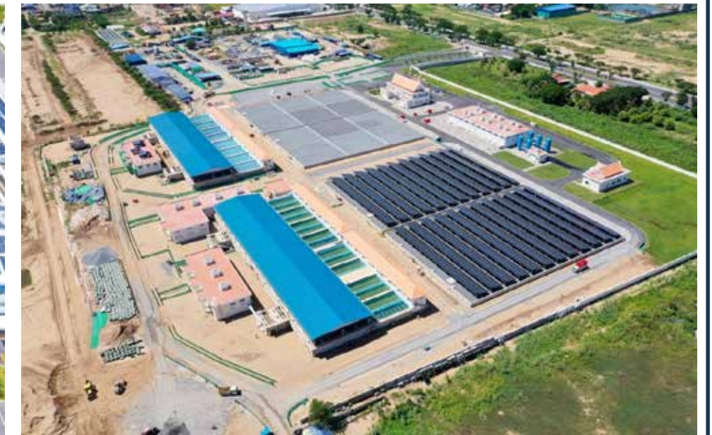
Bakheng Water Treatment Plant
