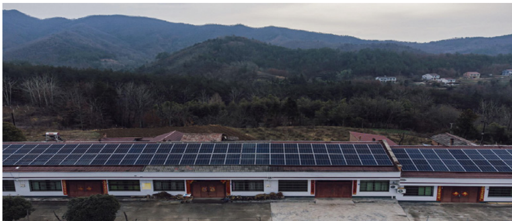
Figure 16: Installation of Solar Panel in Hanyin County.
