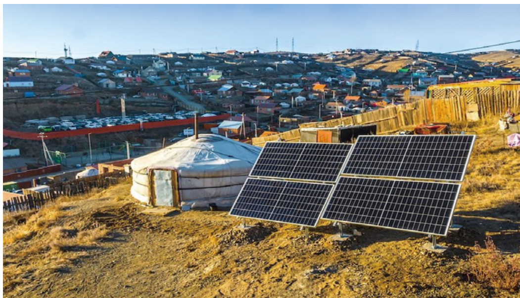
Figure 15: Installation of Solar Panels in Ger District (Source: The Asia Foundation)
